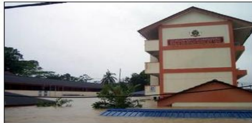
Kota Tinggi, Johor, Jan 14: Sekolah Kebangsaan Bandar is one of the five schools in the district submerged by floodwaters. NST pix by Ahmad Bahri
